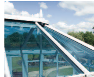
Glass units - reduce solar gain in summer & minimise heat loss in winter with treated glass.
