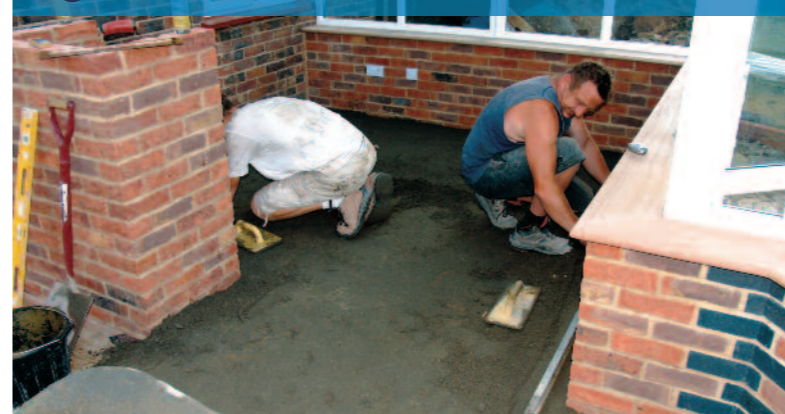
7 Screeding and finishing the floor surface
